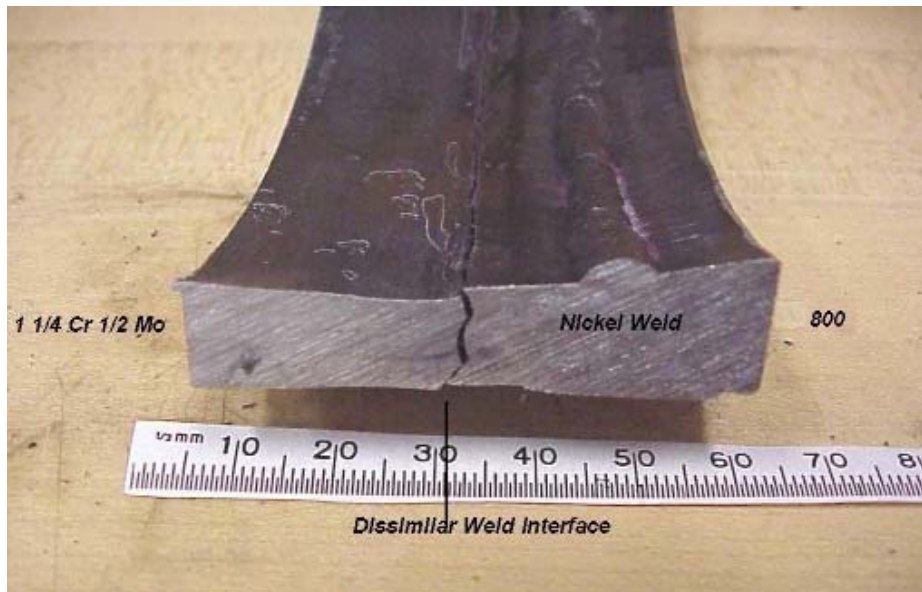
Figure 4-38 – Failure of DMW joining 1.25Cr-0.5Mo to Alloy 800H in a Hydro-dealkylation (HAD) Reactor Effluent Exchanger. Crack propagation due to stresses driven at high temperature of 875°F (468°C) and a hydrogen partial pressure of 280 psig (1.93 MPa).
