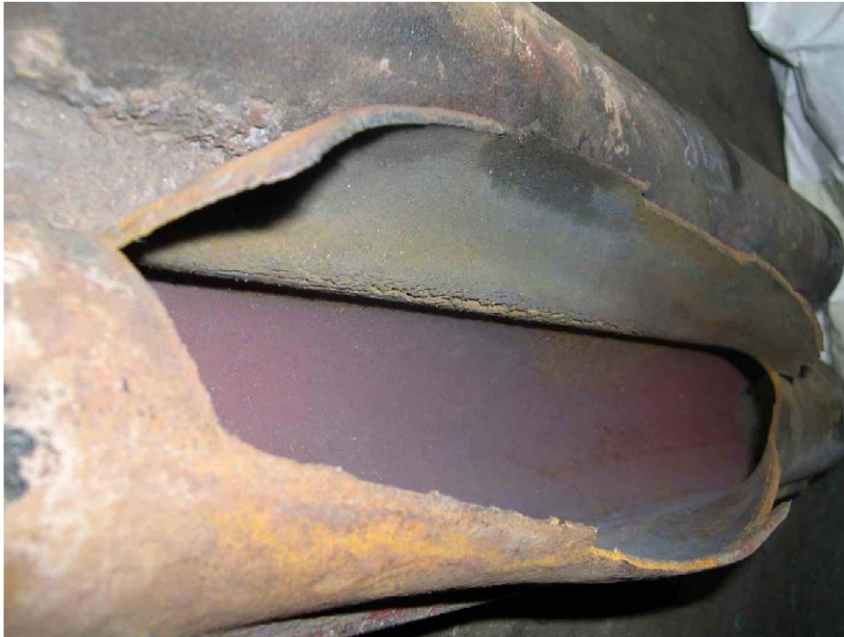
Figure 4-141 – Corrosion fatigue failure of a boiler tube.
