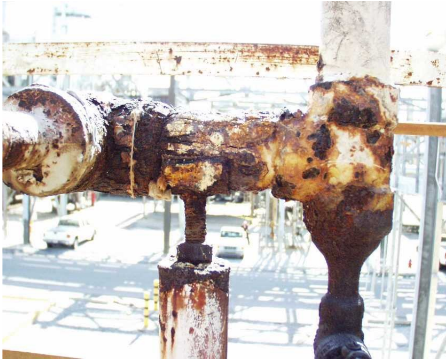
Figure 4-80 – CUI of CS level bridge.
