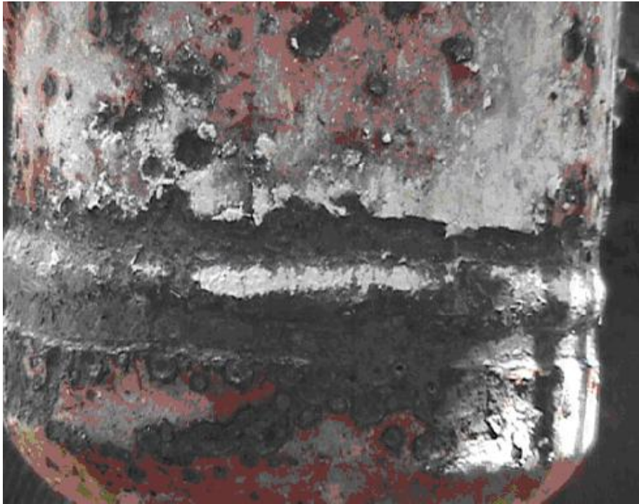
Figure 4-113 – Oxidation of the O.D. of a carbon steel furnace transfer line.
