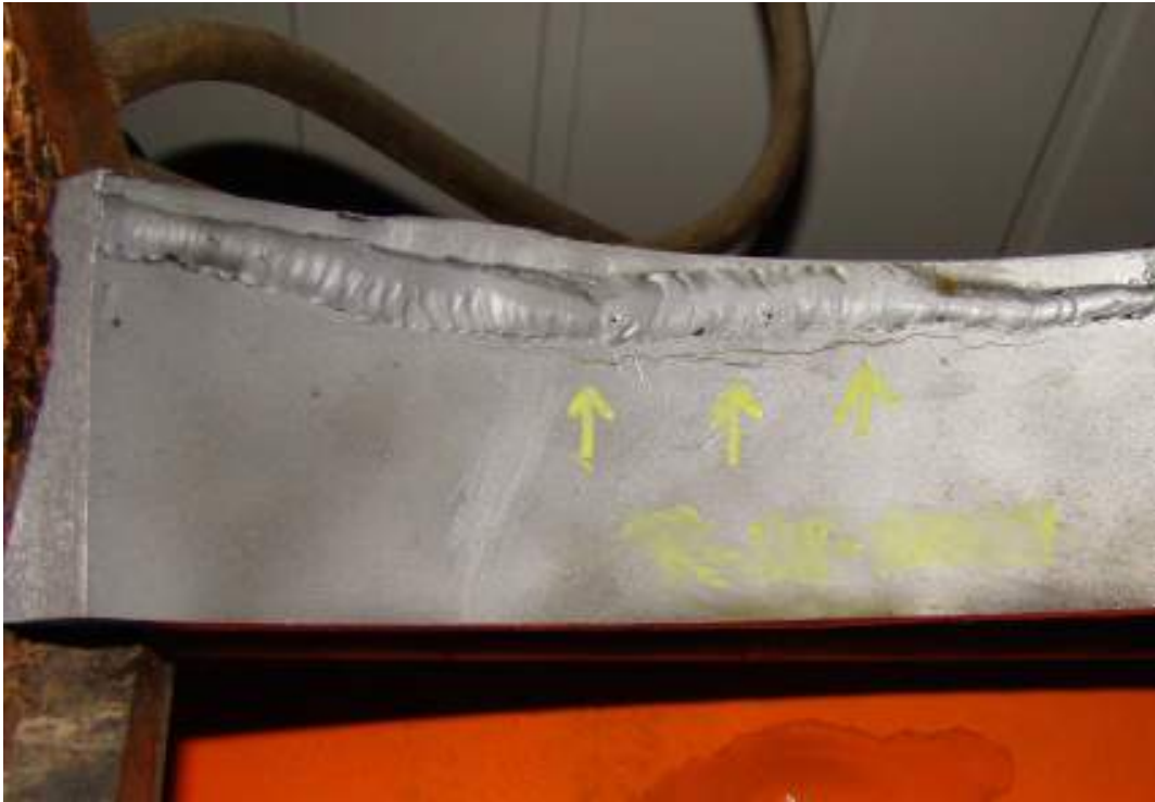
Figure 5-46 – Overhead interstage knockout drum vapor outlet nozzle.
