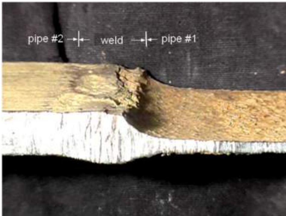
Figure 5-12 – Cross-section of a carbon steel pipe showing preferential corrosion of the pipe with high residual element content on the right, as compared to the low residual pipe section to the left of the weld (Reference 3).
