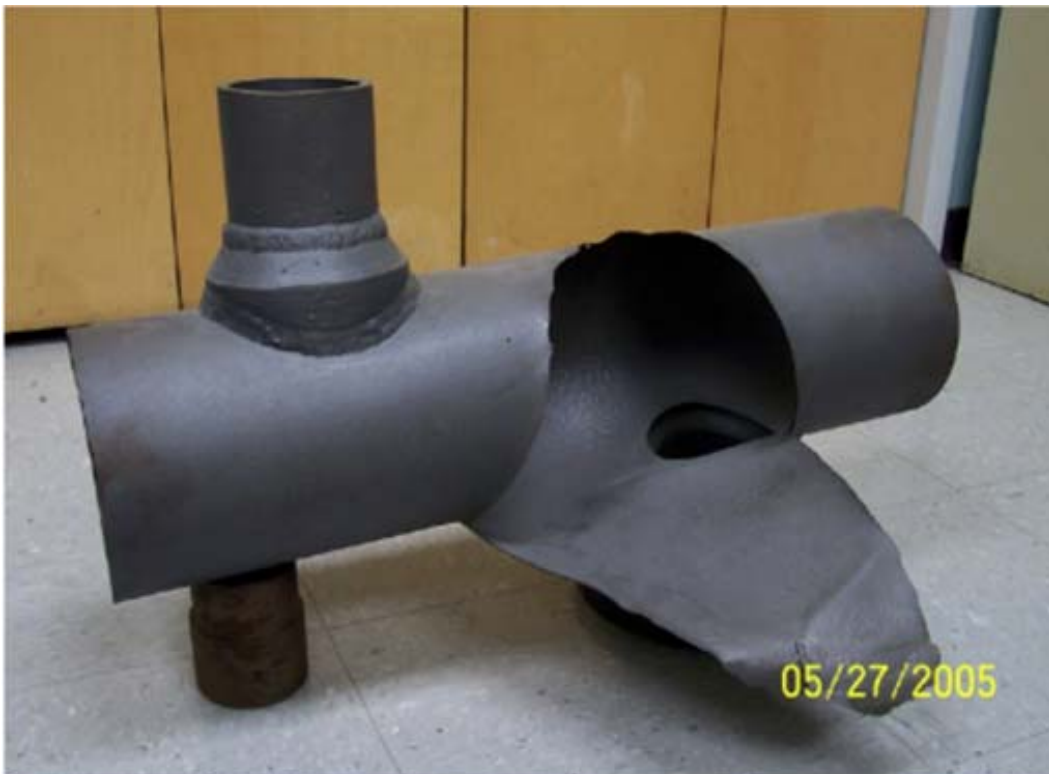
Figure 4-116 – Sulfidation failure of NPS 8 carbon steel pipe. Note the relatively uniform thinning that resulted in a sizeable rupture.
